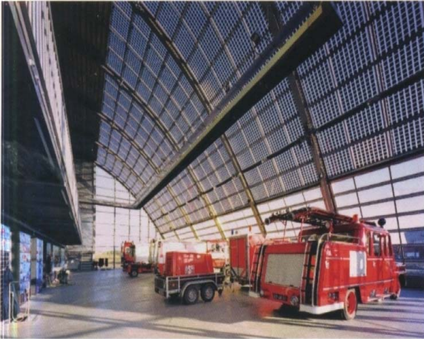
Fig 12 Fire Station Houten, the Netherlands, designed by architect Philippe Samyn
